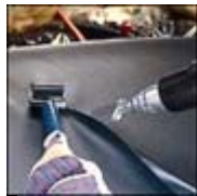
Welding Plastic Materials
